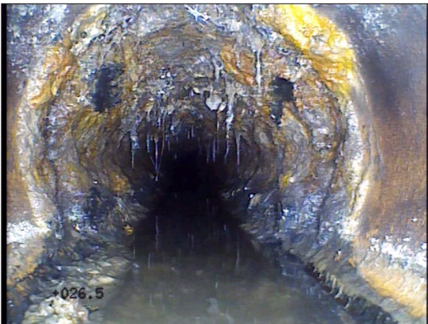
Photo: 38a, Tape No.: 7 25.8m, Encrustation medium, from 07 to 05 o'clock, cross-sectional area loss
