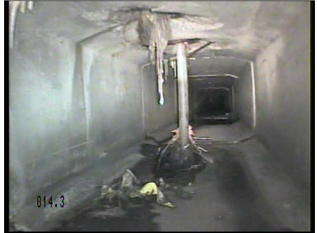
Photo: 16_6a, Tape No.: 1 15.5m, Obstruction, 10 % height/diameter loss
