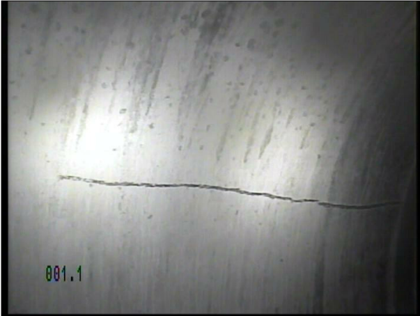
Photo: 17_4a, Tape No.: 1 1.1m, Longitudinal Crack, at 11 o'clock
