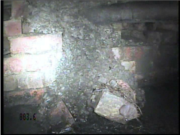
Photo: 2_6a, Tape No.: 1 1.5m, Obstruction, 5 % height/diameter loss
