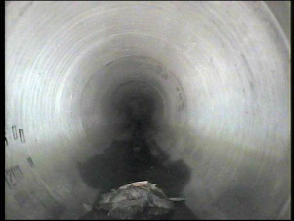
Photo: 15_4a, Tape No.: 1 10.1m, Obstruction, 5 % height/diameter loss
