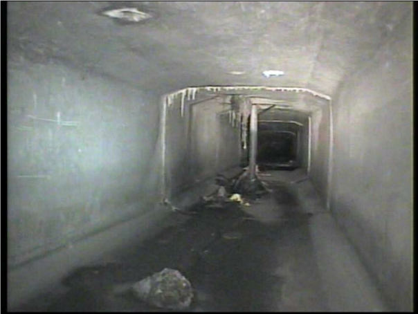
Photo: 16_5a, Tape No.: 1 12.8m, Obstruction, 5 % height/diameter loss
