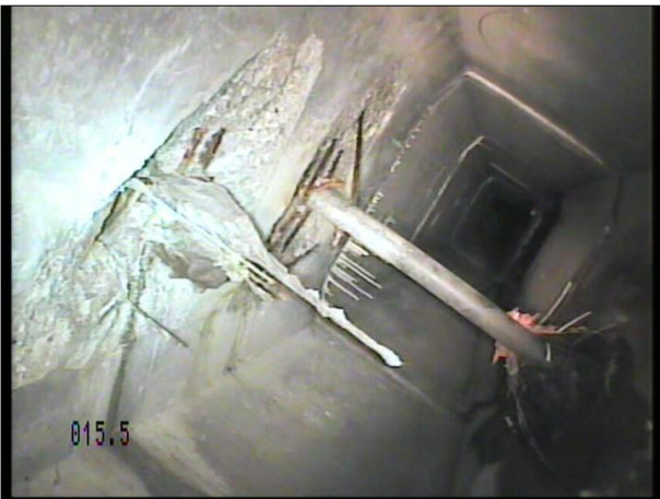
Photo: 16_7a, Tape No.: 1 15.5m, Surface damage, spalling medium, at 12 o'clock
