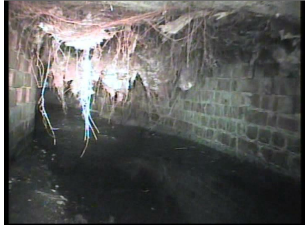
Photo: 2_15a, Tape No.: 1 23.5m, Mass Roots 10 % cross-sectional area loss
