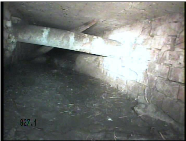
Photo: 2_18a, Tape No.: 1 28.2m, Connection, at 10 o'clock, dia 150 mm. Enclosed Pipe
