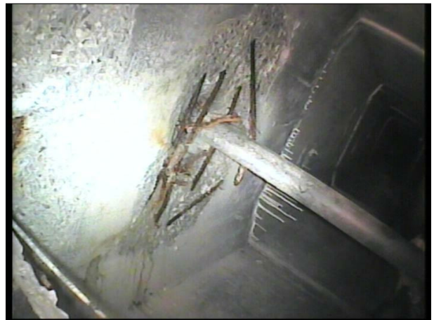
Photo: 16_7b, Tape No.: 1 15.5m, Surface damage, spalling medium, at 12 o'clock
