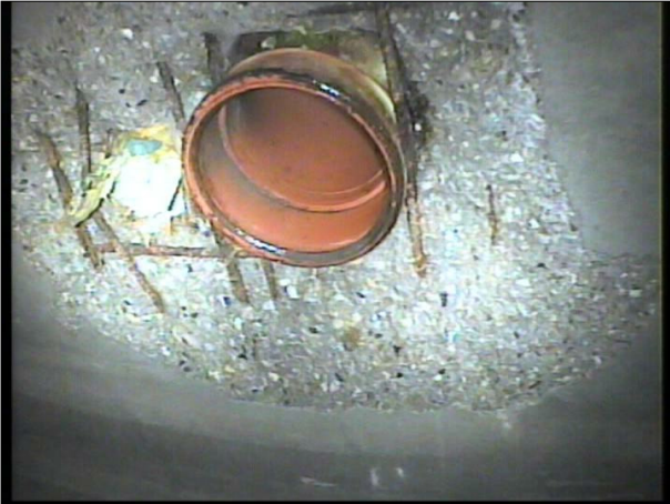
Photo: 9_6a, Tape No.: 1 3.7m, Surface damage, spalling slight, from 12 to 01 o'clock
