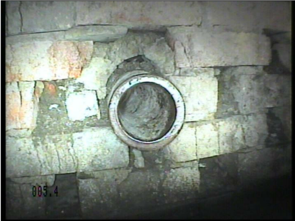
Photo: 8_6a, Tape No.: 1 5.4m, Connection, at 09 o'clock, dia 100 mm, intrusion 50 mm
