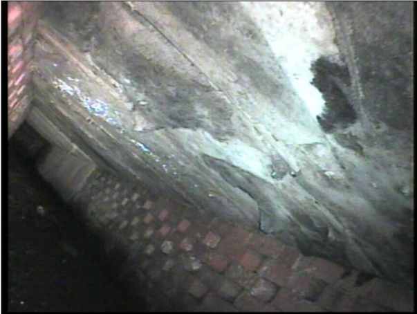
Photo: 3_8a, Tape No.: 1 18.1m, Surface damage wear from 10 to 02 o'clock
